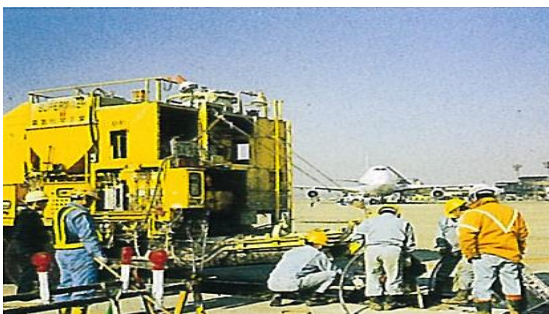
Repairing for apron of Airport
