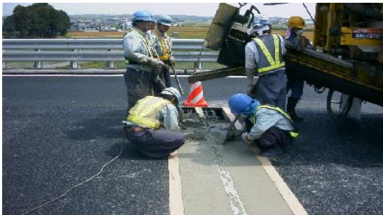
Repairing for expansion joint of Bridge
