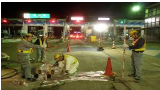
Repairing for Tollgate of Highway
