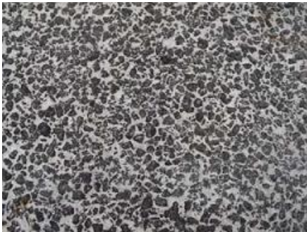
Semi-rigid pavement with asphalt
